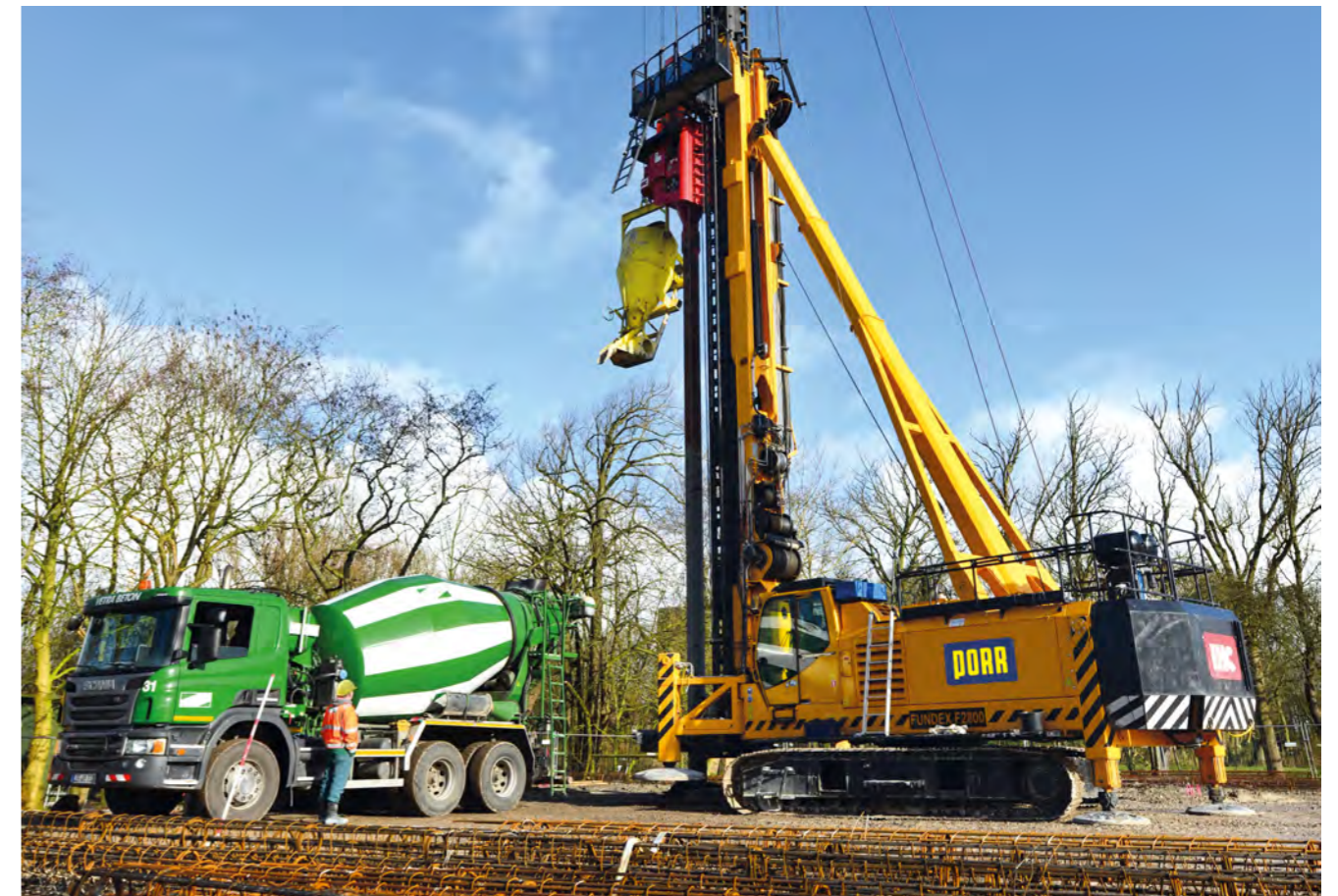
Making Fundex piles in Wangerland
