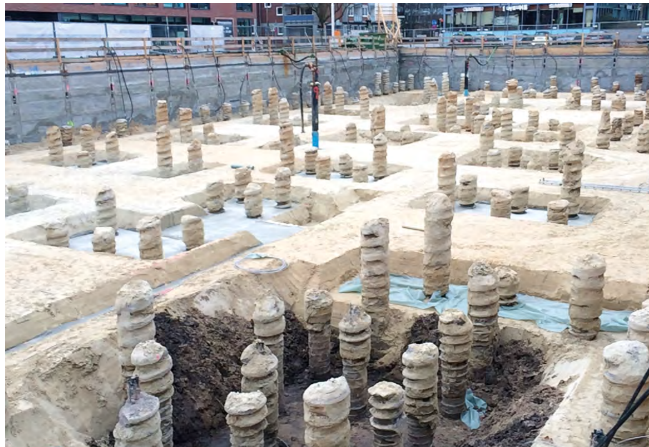
Exposed Atlas piles before capping
