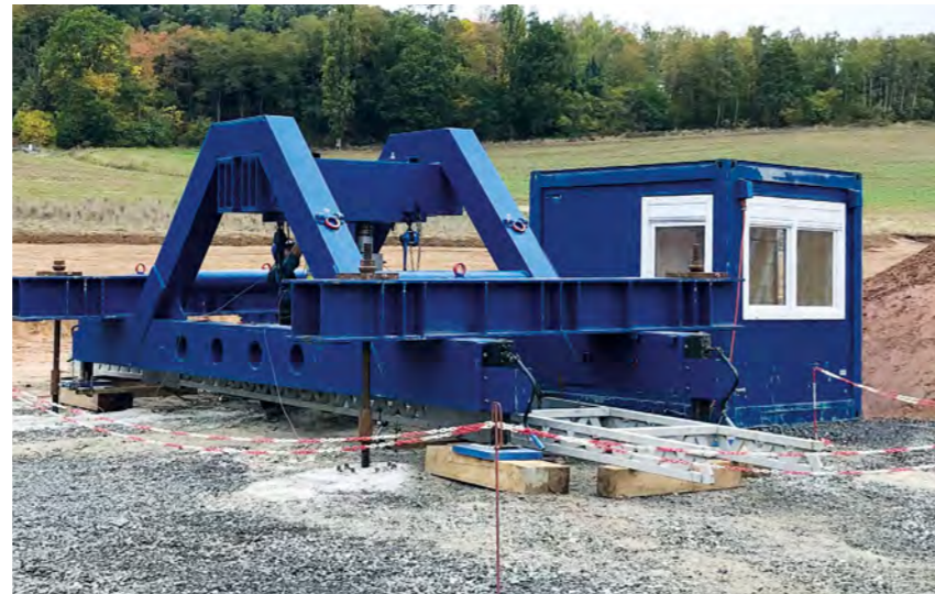
Static pile load test
