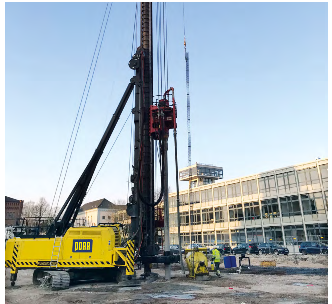
Production of Atlas piles in Oldenburg
