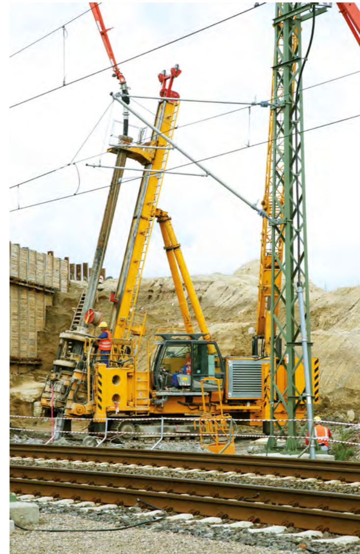
Vibration-free execution with Atlas piles next to railway tracks.
