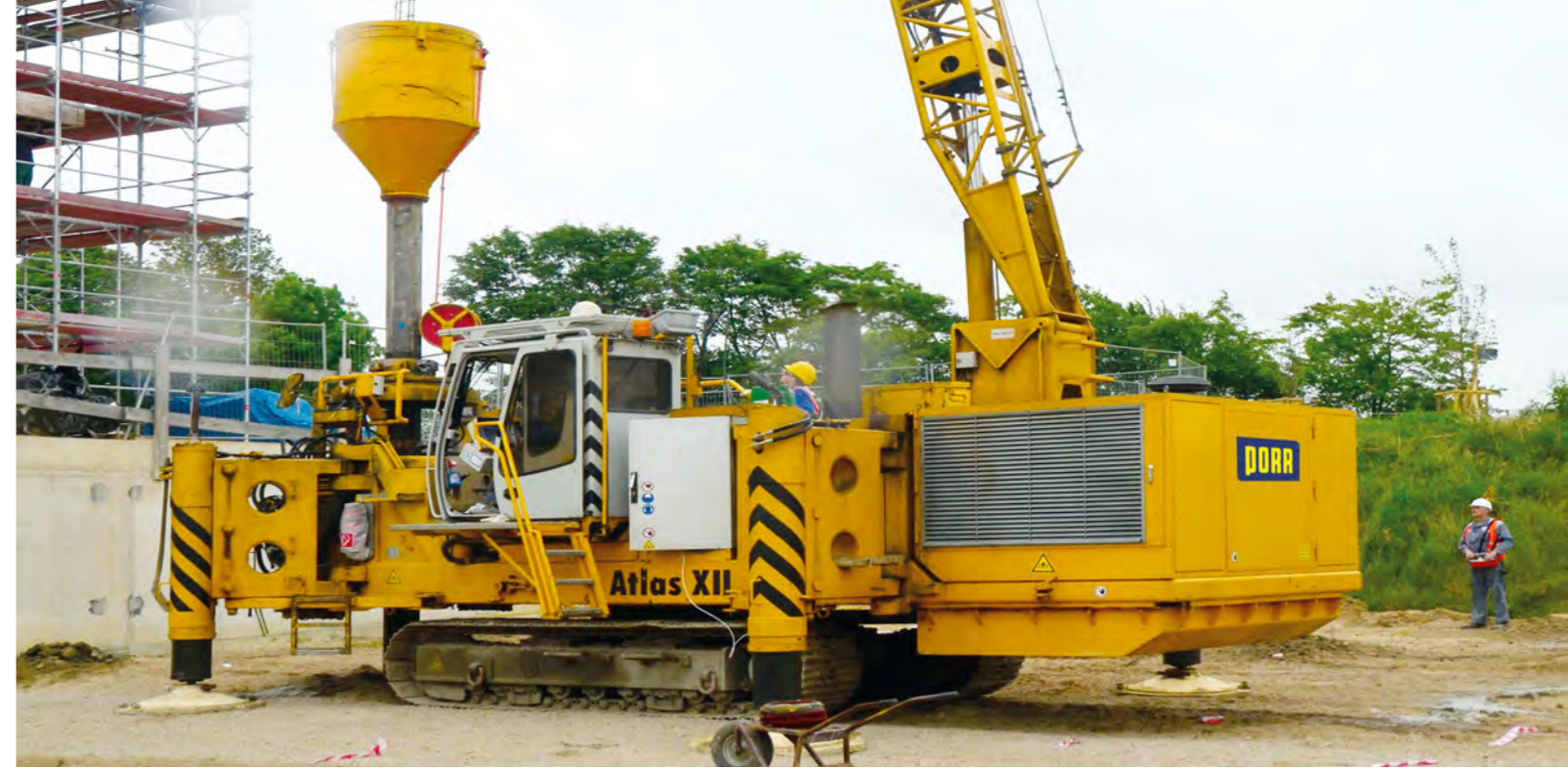
Adjusting a reinforcement cage for the atlas pile
