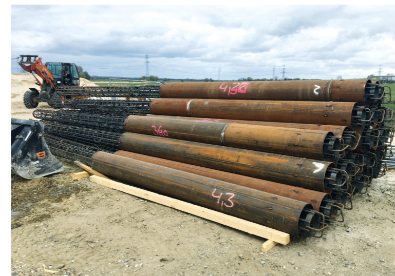
Frankipiles NG® for the bridge on the BAB 26. In the area of the peat layers, sleeves were required for the to support the fresh concrete columns.
