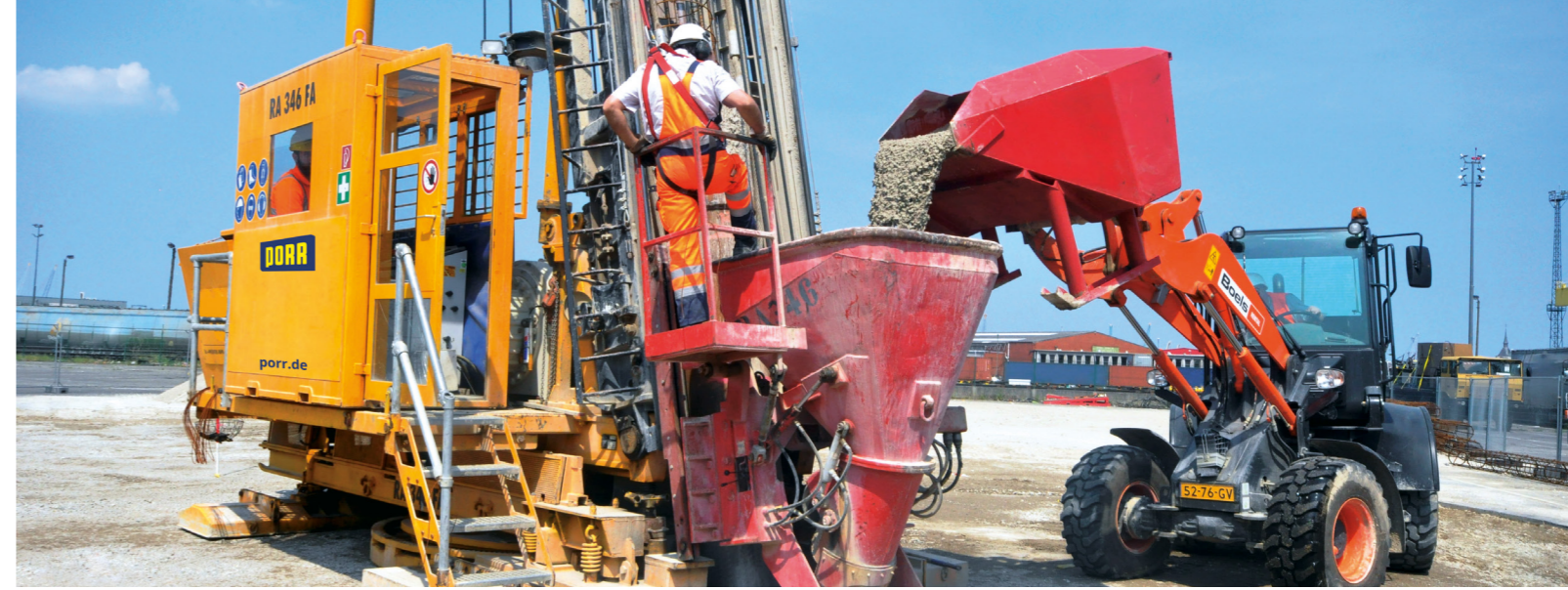
Concreting a Frankipile NG®
