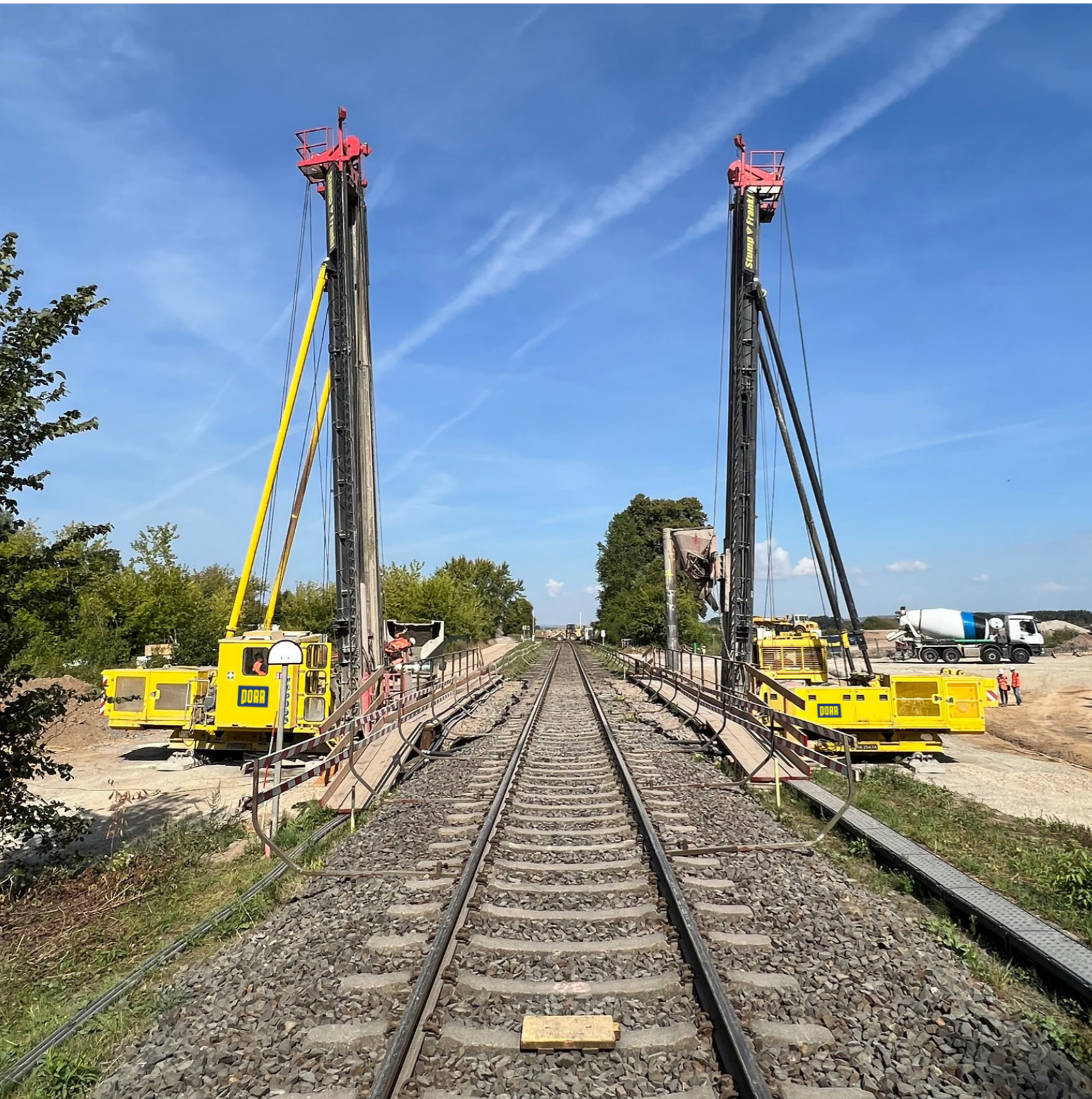
Mühlhausen bypass. Frankipile NG® next to railway tracks..
