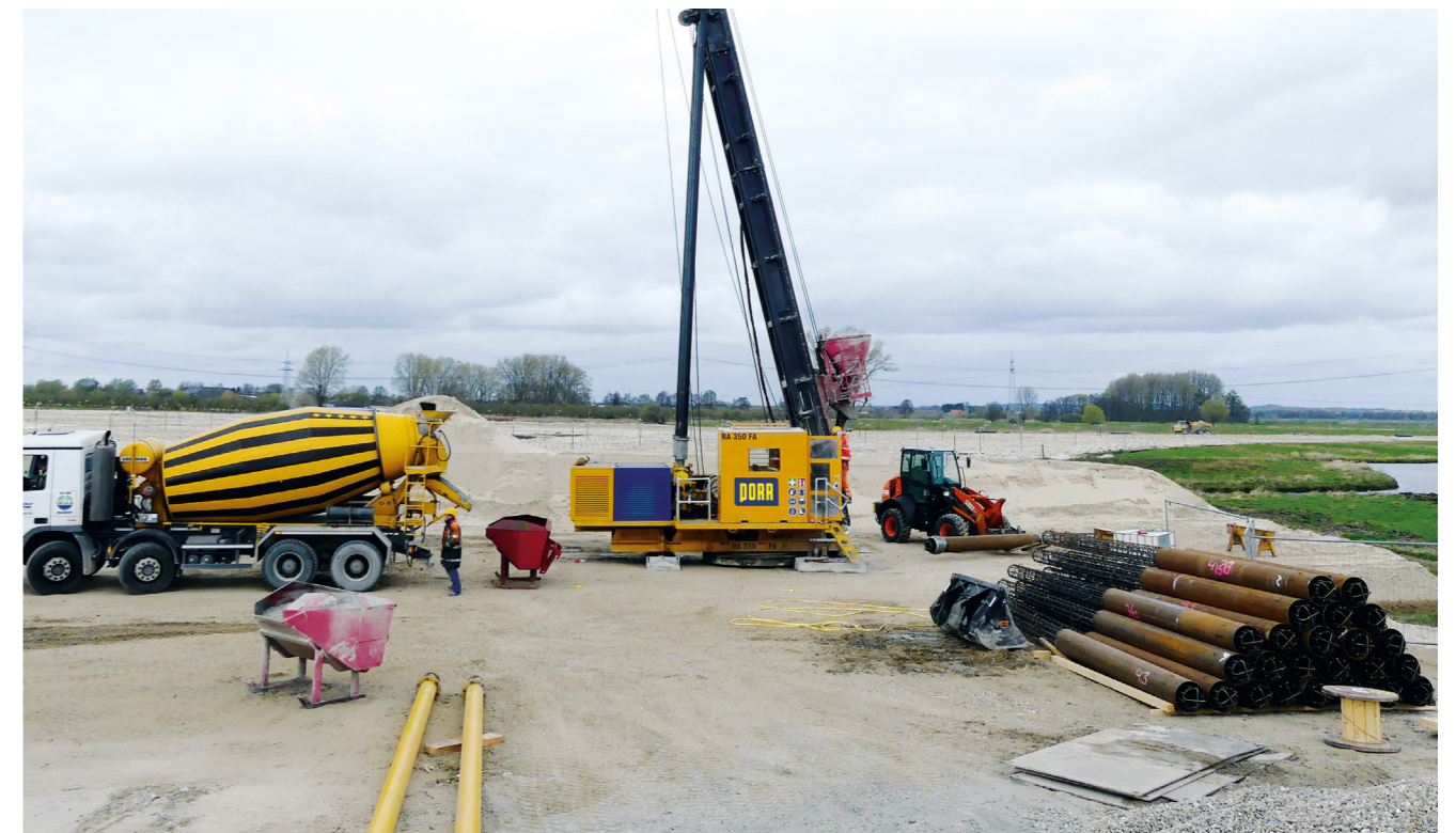
Frankipiles NG® for the bridge on the BAB 26. In the area of the peat layers, sleeves were required for the to support the fresh concrete columns.
