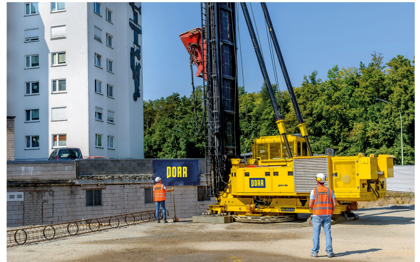
Construction of Frankipiles NG® next to an existing building
