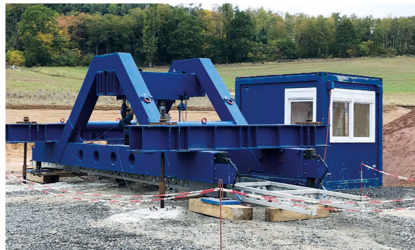
Static pile load test
