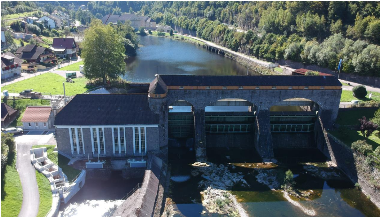
Rudolf Fettweis Plant in Forbach © EnBW, Ingo Kamuf
